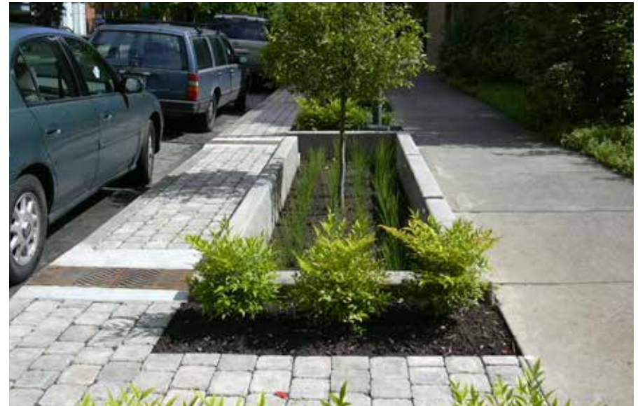
Examples of infiltration and flow-through planters
