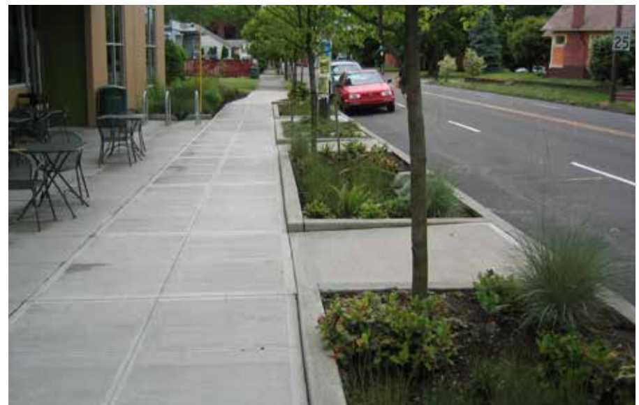
Examples of infiltration and flow-through planters
