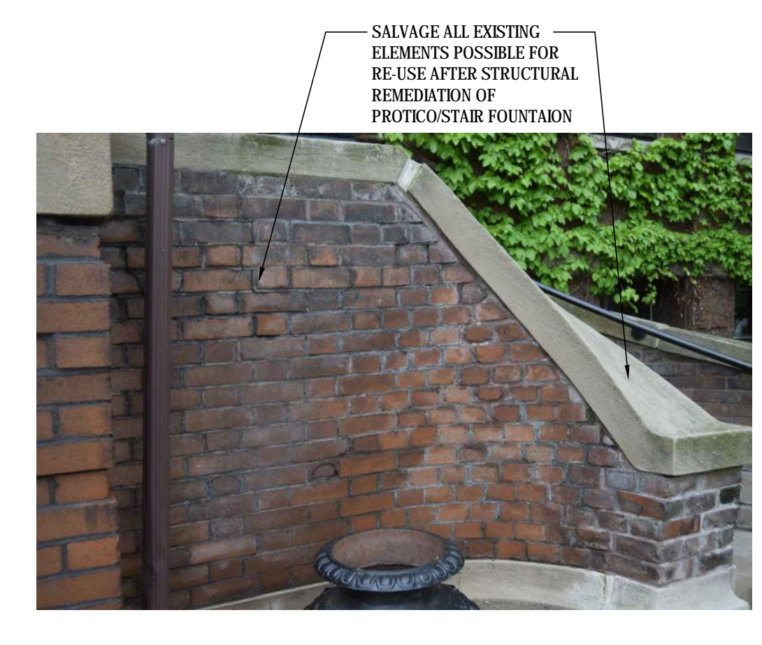
14 A401 DETAIL OF EXCHANGE STREET STAIR NO SCALE
