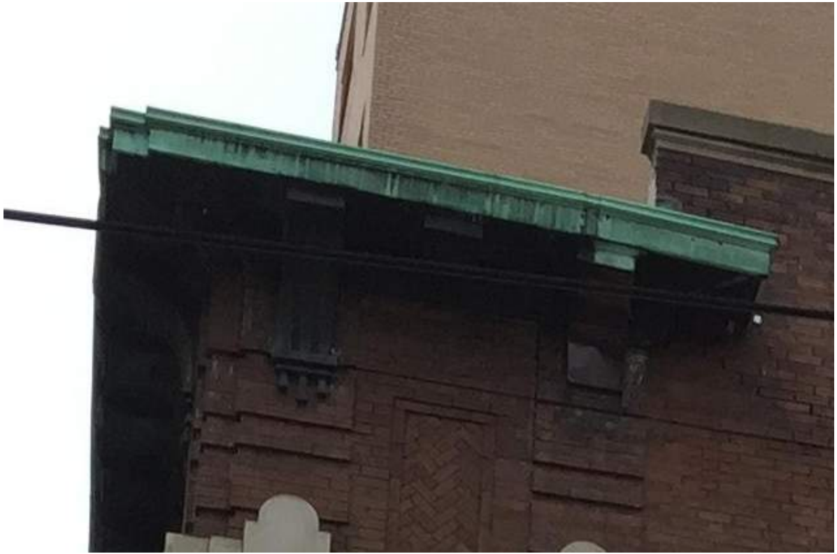
cedar street side - south building
