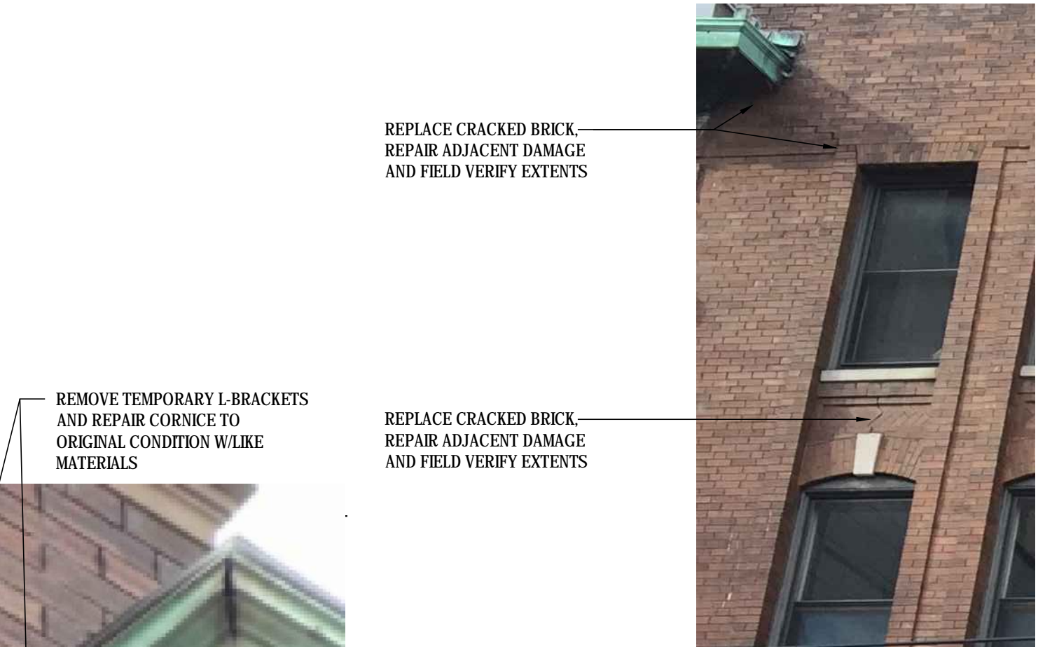
PHOTO AT DAMAGED MASONRY NO SCALE
