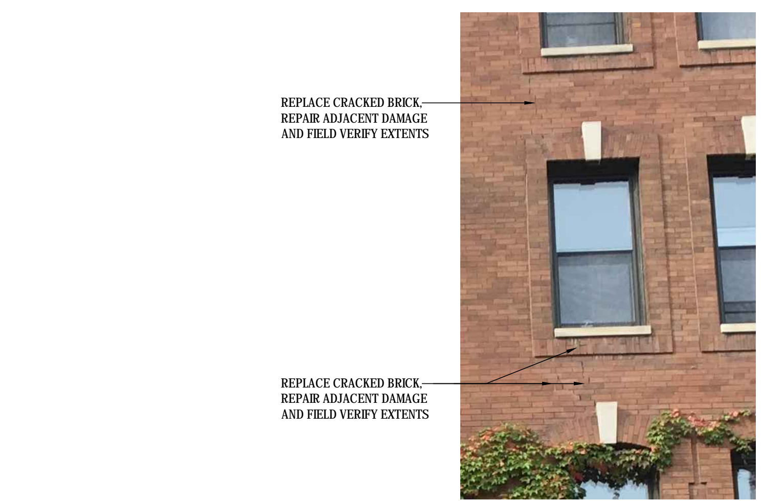
PHOTO AT CRACKED MASONRY NO SCALE
