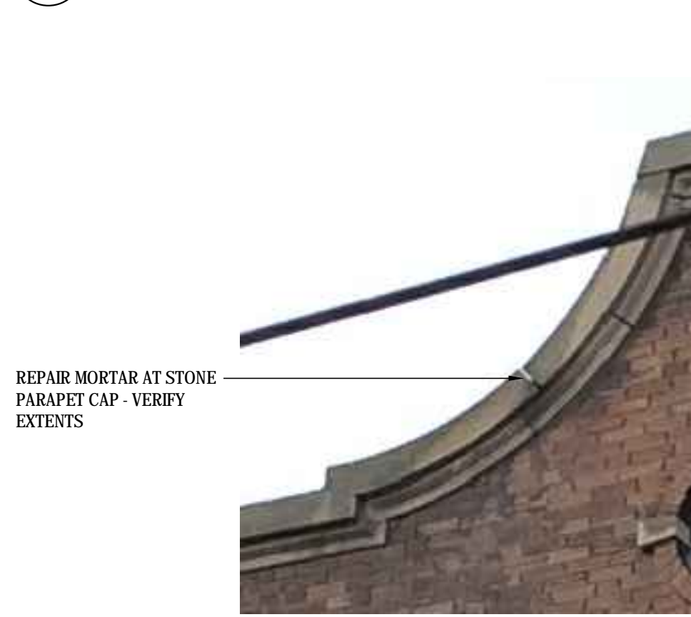
REPAIR MORTAR AT STONE PARAPET CAP - VERIFY EXTENTS
