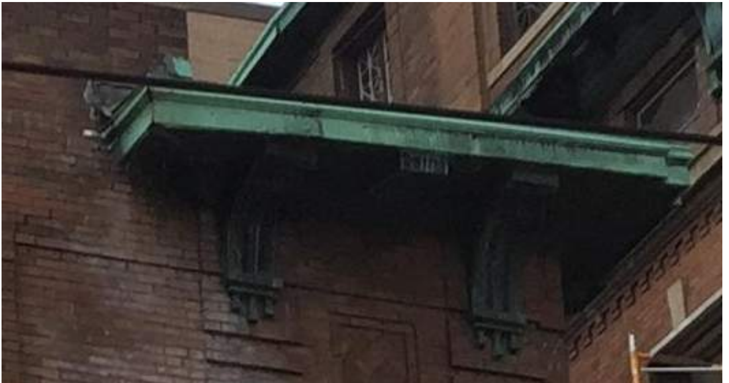
cedar street side - south building
