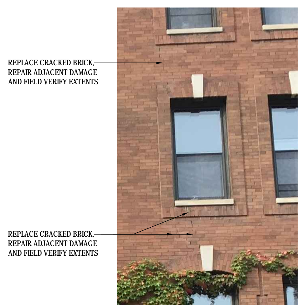
PHOTO AT CRACKED MASONRY NO SCALE
