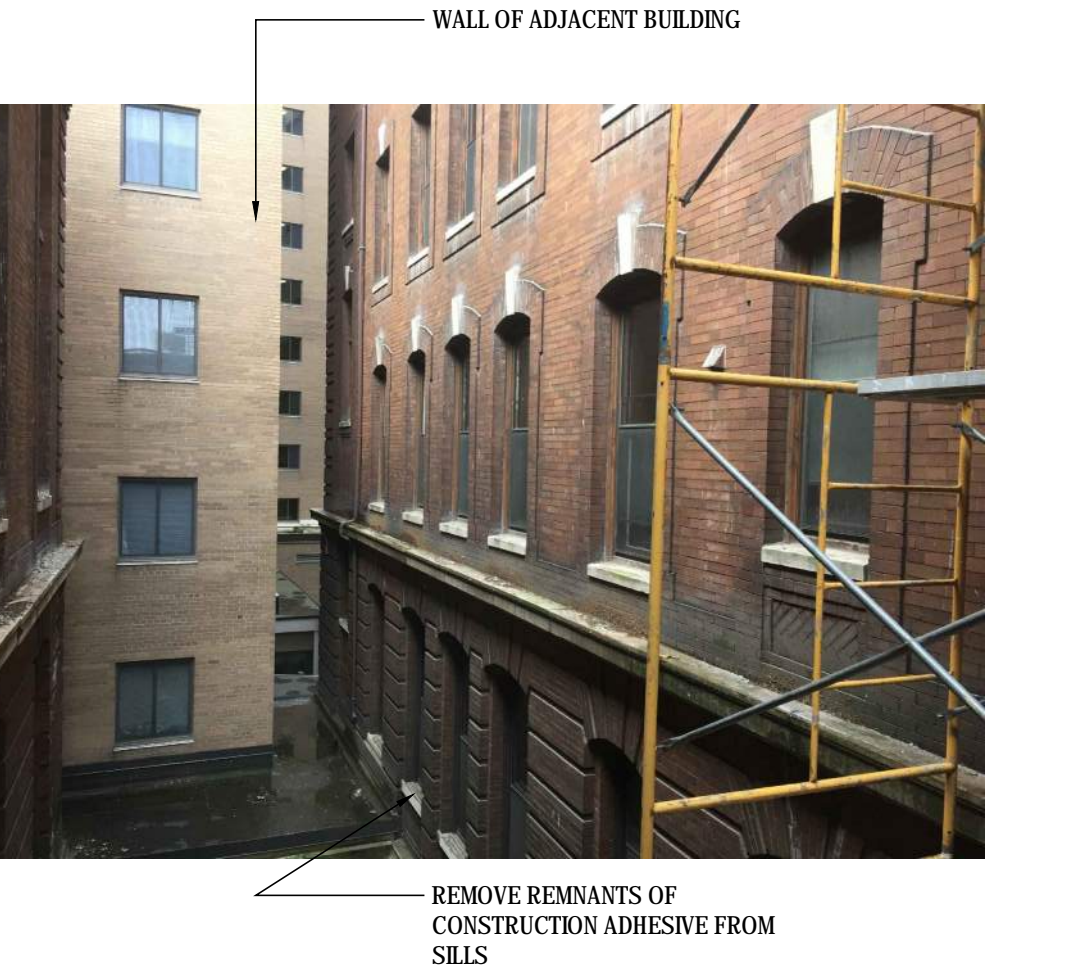
8 A401 VIEW OF COURTYARD SIDE OF NORTH BUILDING NO SCALE
