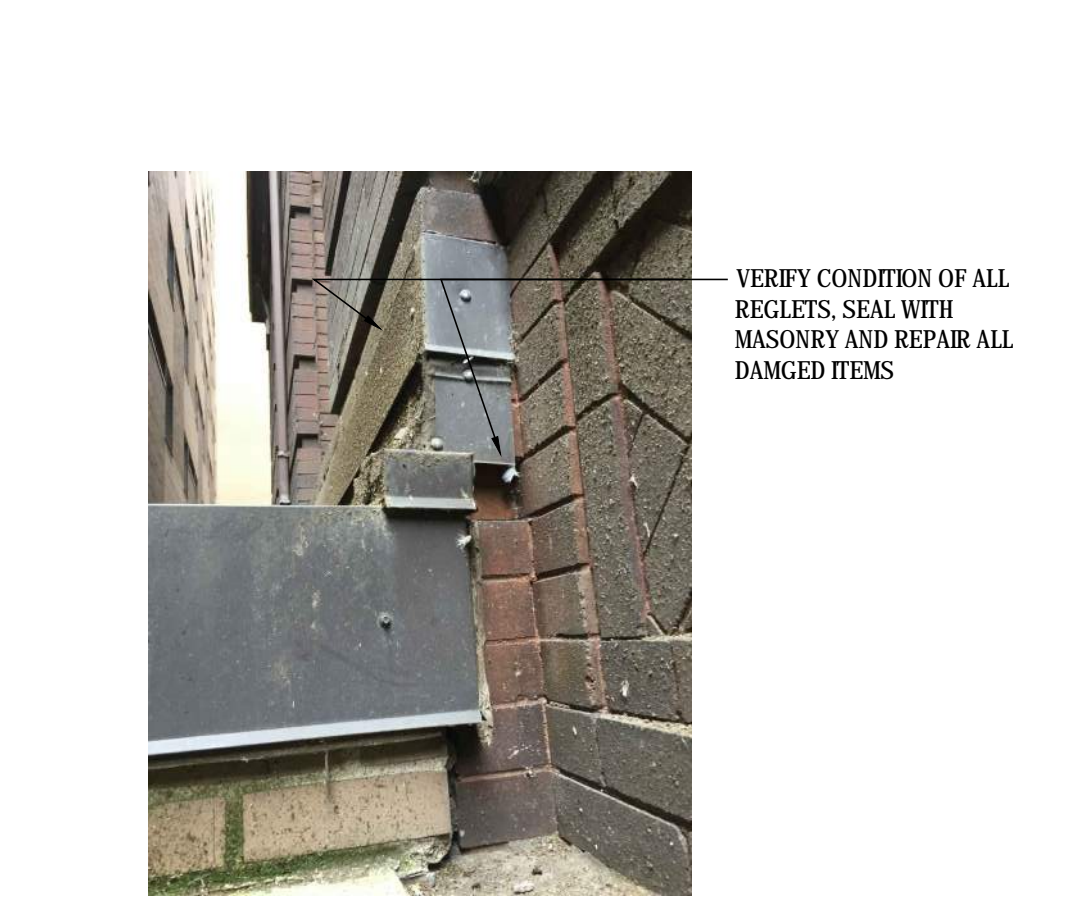
13 A401 FLASHING DETAIL IN COURTYARD NO SCALE
