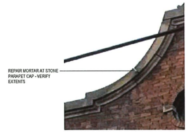
19 A400 PHOTO AT SOUTH BUILDING PARAPET NO SCALE
