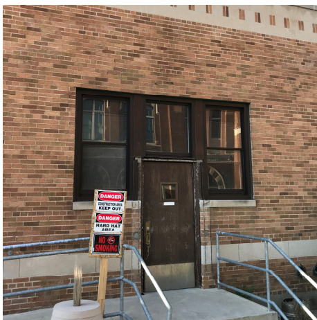
South façade door to be expanded
