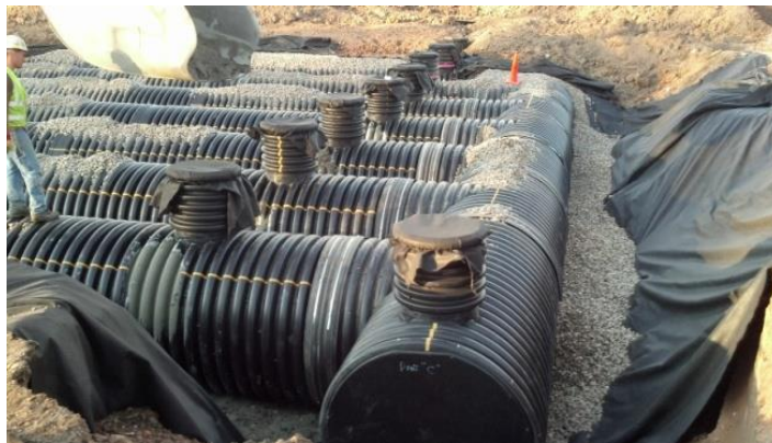
Photo 4-1: 60" Perforated HDPE pipes during system construction
