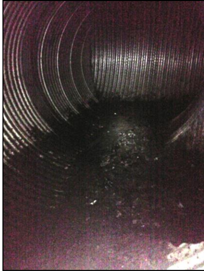
Photo 6-1: Underground perforated CMP storage chambers
