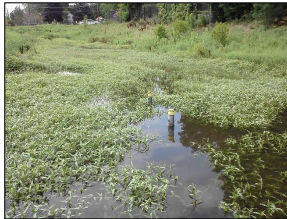
Photo 3-2: Infiltration basin located above storage chambers
