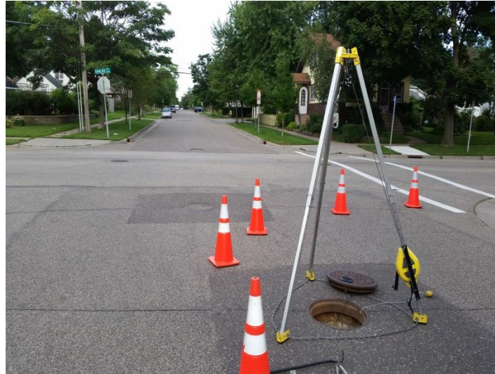
Photo 6-2: Accessing flow meters installed in the AHUG diversion structure.
