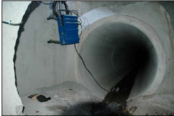
Photo 2-2: Flow module in Beacon Bluff diversion structure (looking upstream)
