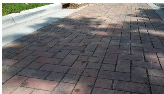
Photo 12-1: Interlocking Pavers at Victoria Street
