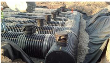
Photo 4-1: 60" Perforated HDPE pipes during system construction
