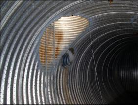
Photo 3-1: Underground perforated storage chambers and access port
