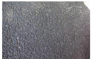
Photo 11-4: Silt accumulation on Hamline Midway Library asphalt (2015).
