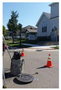
Photo 5-2: Saint Albans water quality sampler at the BMP diversion structure
