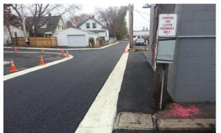
Photo 11-3: Recently Constructed Hamline Midway Library Porous Asphalt (2012)
