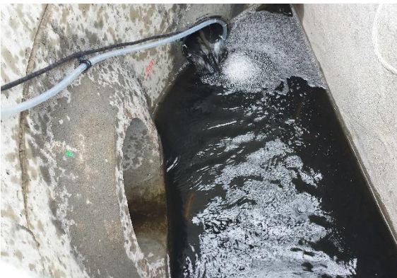
Photo 2-5: Jenks Pond 8" drain tile and outlet pipe within the outlet control structure
