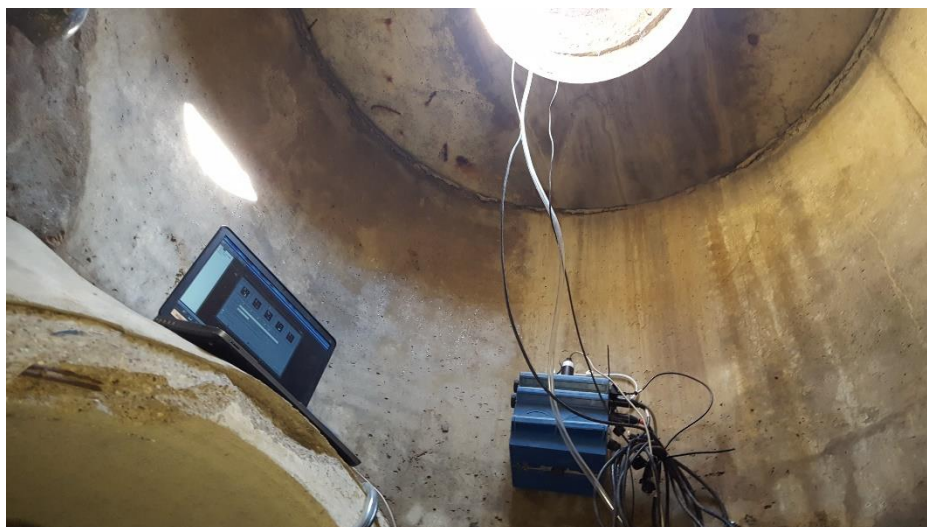
Photo 9-1: Robie Street Flow Meter Installation
