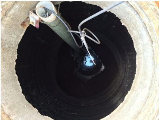
Photo 2-1: Infiltration gallery level monitoring enclosure
