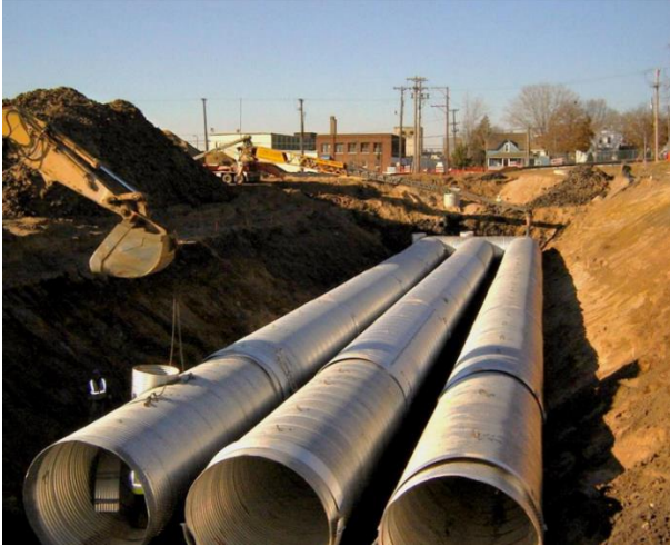
Photo 4-1: Underground infiltration chamber (Facing west)
