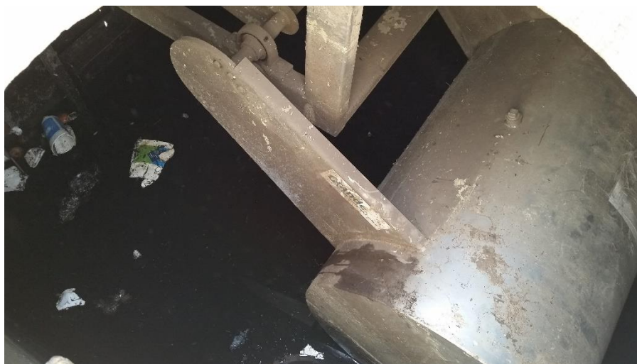
Photo 5-3: System gate valve and float
