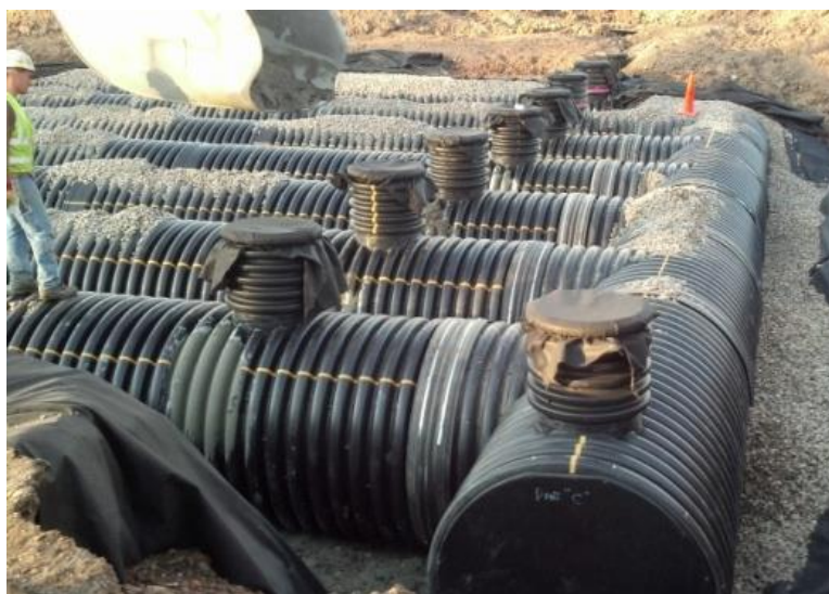
Photo 5-2: 60" Perforated HDPE pipes during system construction
