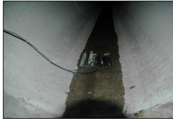
Photo 2-4: Flow sensor in upstream pipe in Beacon Bluff diversion structure
