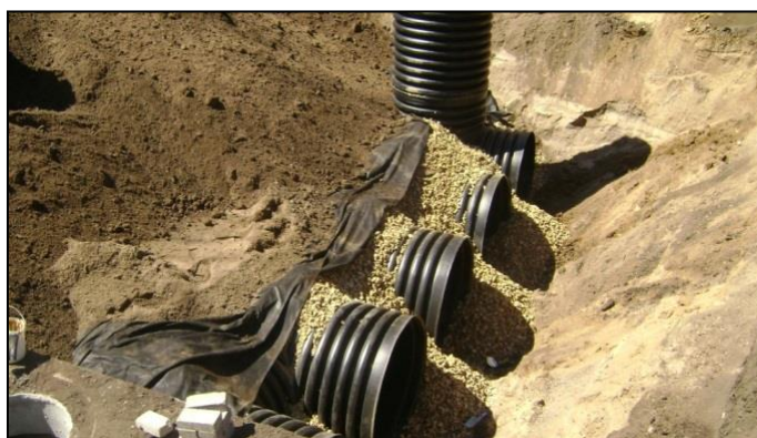
Photo 6-1: St. Albans 48" perforated HDPE installation
