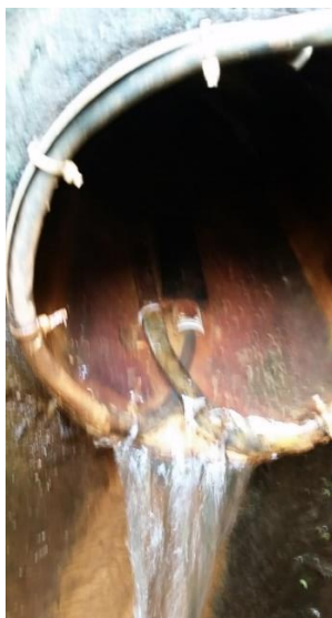
Photo 10-5: Iron Precipitate at drain tile outlet to OCS
