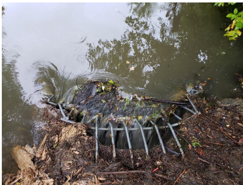
Photo 8-1: Debris in Battle Creek 72" Arch RCP pipe
