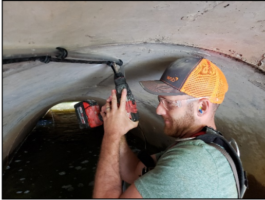
Photo 2-3: Flow Monitoring Module Install Process
