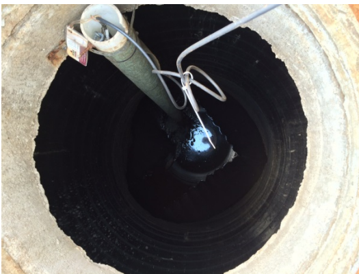
Photo 2-1: Infiltration Gallery Level Monitoring Enclosure
