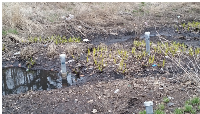
Photo 2-2: Beacon Bluff Rain Garden and In-Rock Wells
