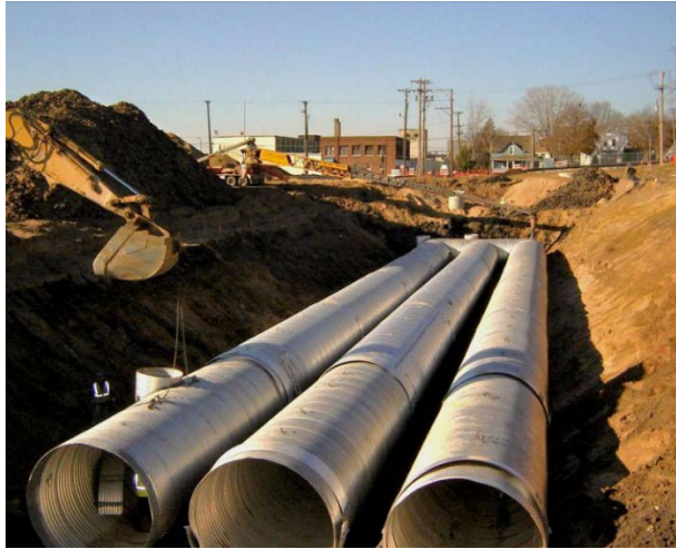
Photo 4-1: Underground Infiltration Chamber (Facing West)
