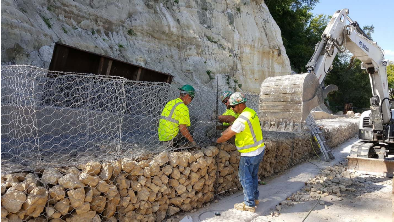
Figure 3. Building a level and stable gabion wall requires care, and a lot of wire.
