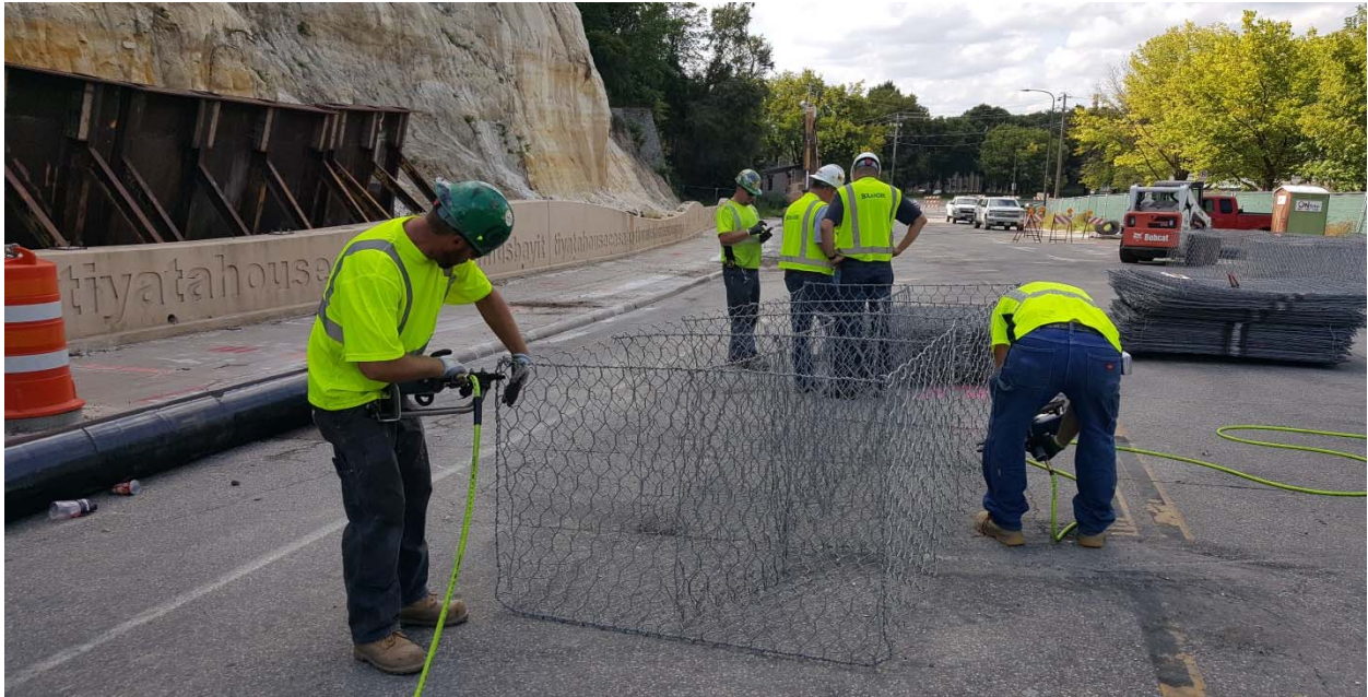
Figure 1. Crews review the material delivery and wall plans, and begin assembly.
