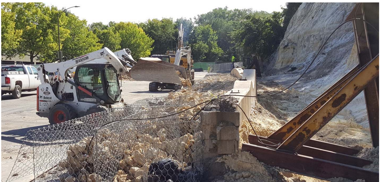
Figure 4. Rock-filling nears the end; crews begin placing a 2 nd layer of baskets.
