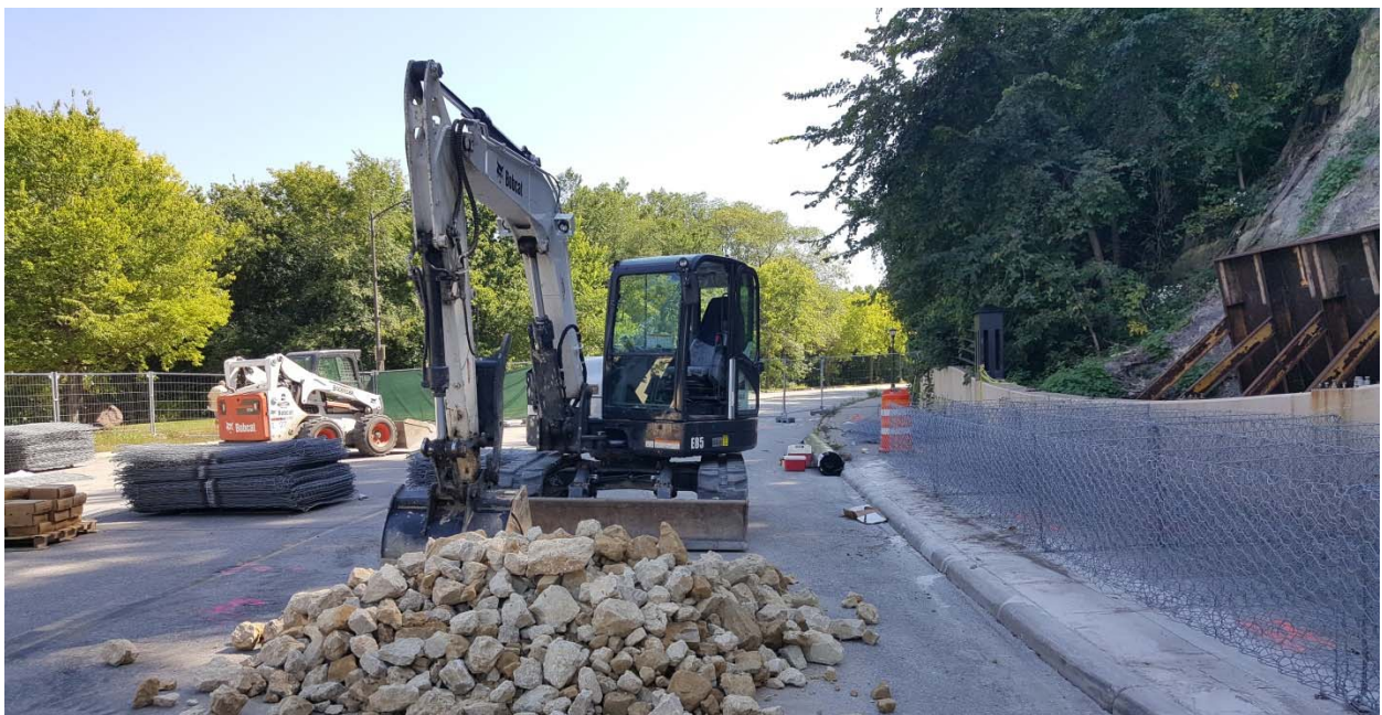
Figure 2. The first course of baskets are set in place and ready to fill with rock.
