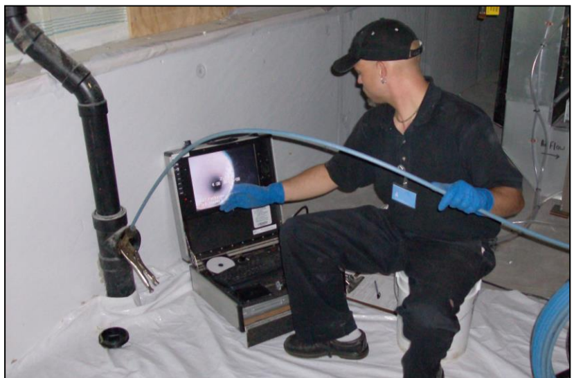
Televised scoping through the vertical cleanout access in sewer pipes. Watch a video at https://youtu.be/SmL8PPJhpiw
