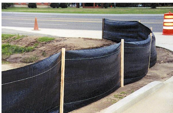
Properly installed silt fence
