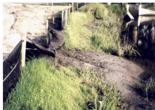
Silt fence that was not maintained
