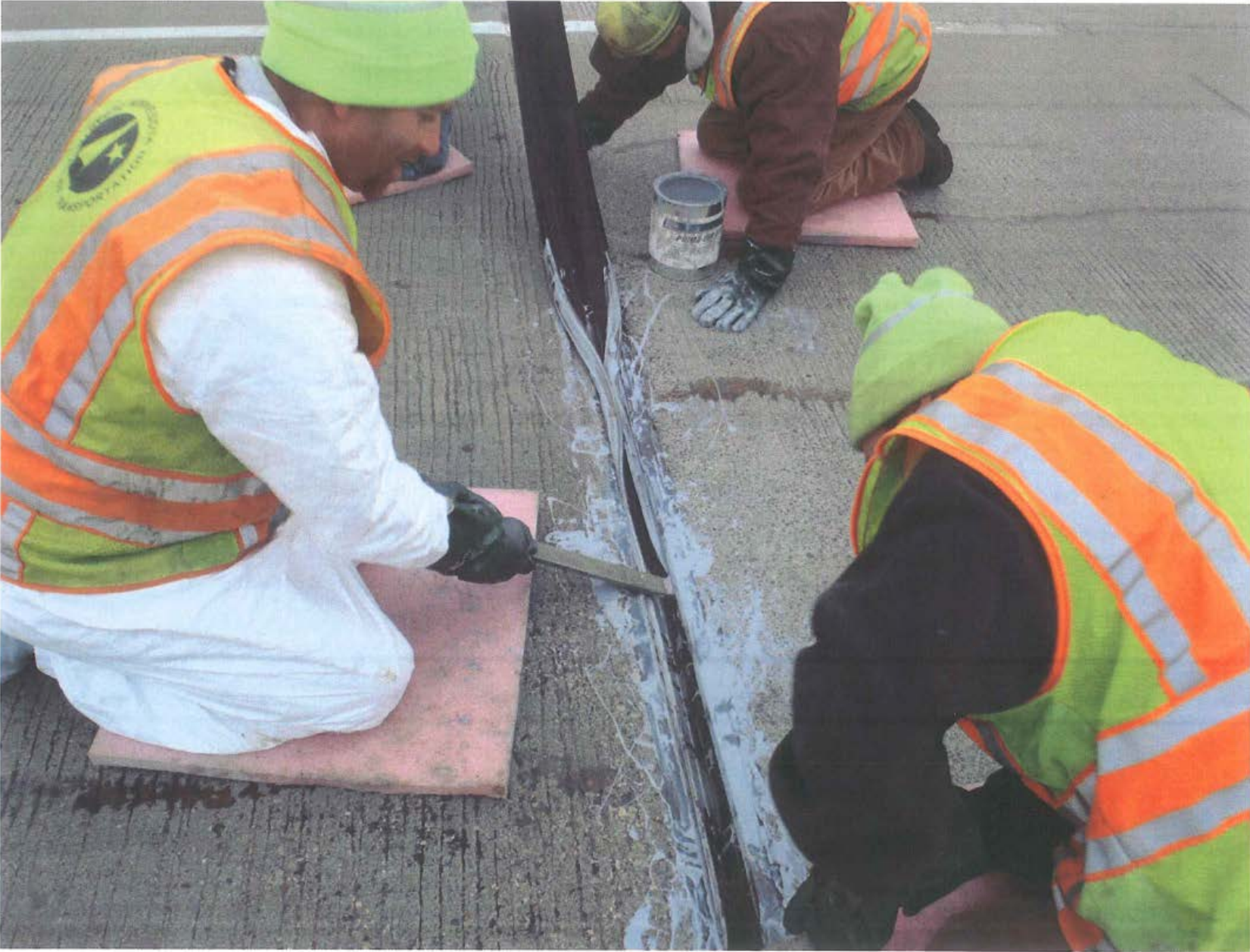
Sample Photo of Gland Installation
