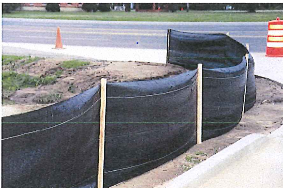
Properly installed silt fence
