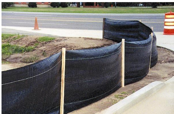
Properly installed silt fence
