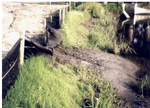
Silt fence that was not maintained
