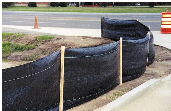
Properly installed silt fence
