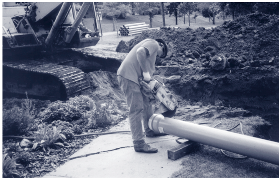
Staff installing various types of pipe.
