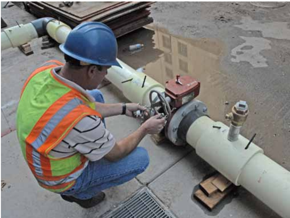
Checking a valve on a temporary water main providing water to a downtown office building in conjunction with the light rail utility relocation work.
