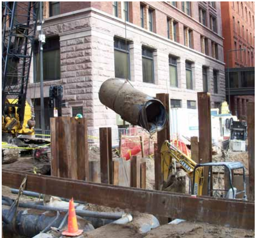
Photos opposite: Top, engineers check the site plans for Sandy Lake. Bottom, the demolition of the Dale Street reservoir to make room for the new reservoir. This page, above, work replacing water main on the Central Corridor-Light Rail Transit project in downtown Saint Paul.
