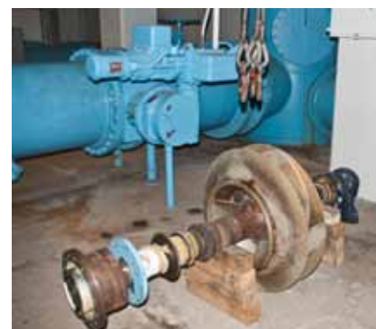
Photo above: Pump No. 5 at the Fridley pumping station has reached the end of its useful life and will be replaced.
