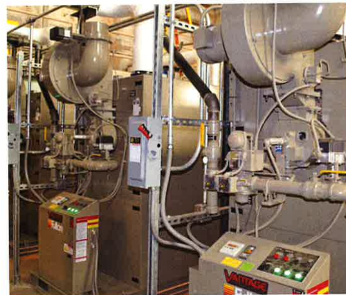
Pleasant Lake oxygenation system (top). Pump No. 5 at the Fridley station (middle). Newly installed boilers (bottom).
