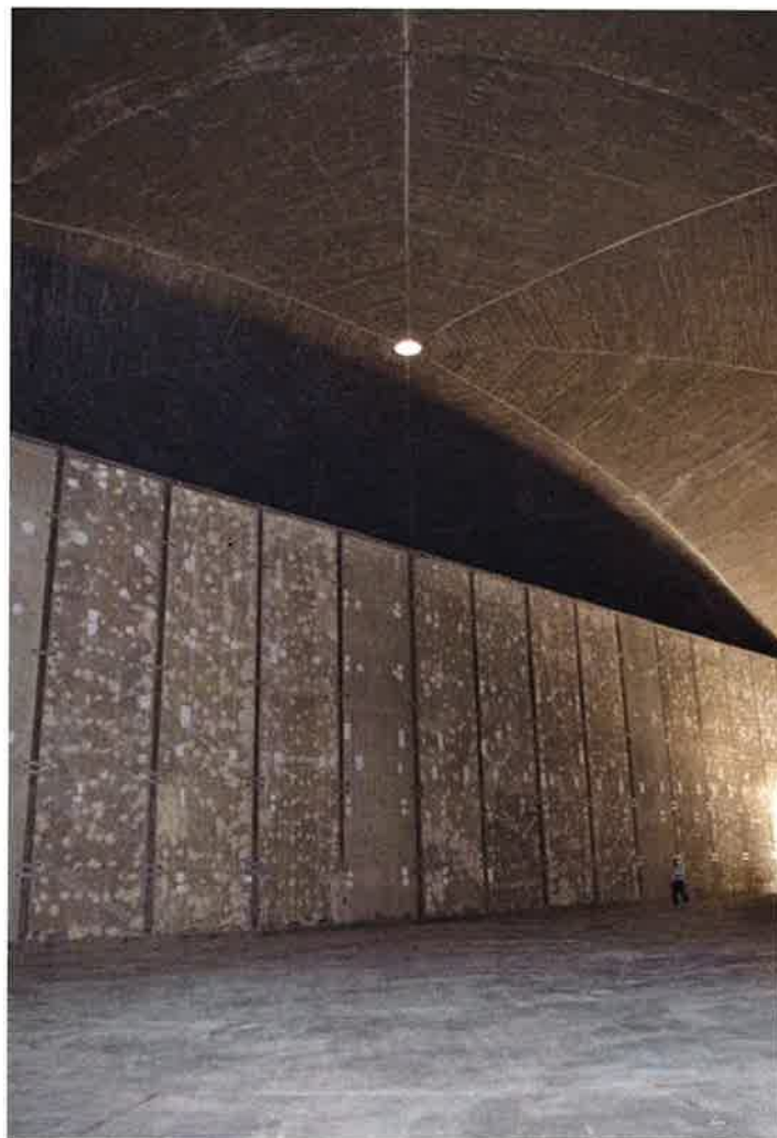
Inside the 10-million-gallon reservoir at Roseville, which replaces the old reservoir.
