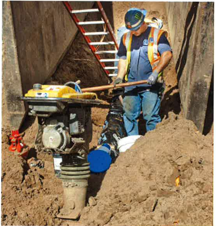
Workers replace a water main (above). Replacing the sidewalk after work is complete (opposite).
