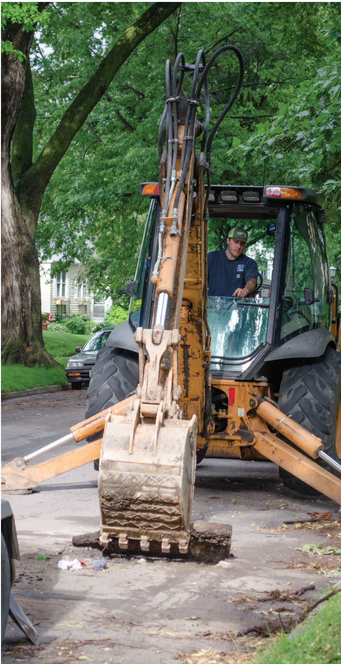
A worker opens the street in preparation for a partial lead service line replacement. SPRWS did 406 partial lead service line replacements in 2016.
