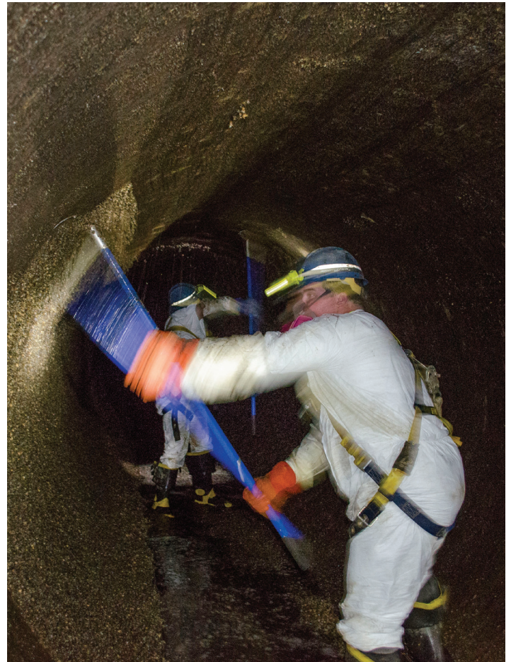
Workers remove zebra mussels from the Vadnais conduits.
