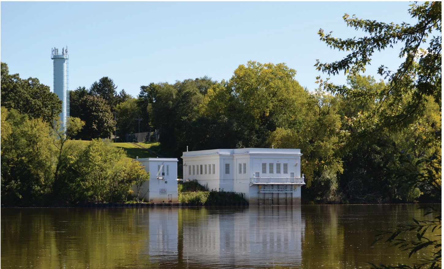
The Mississippi River pumping station in Fridley was built in the early 1920s and put into service in 1925.
