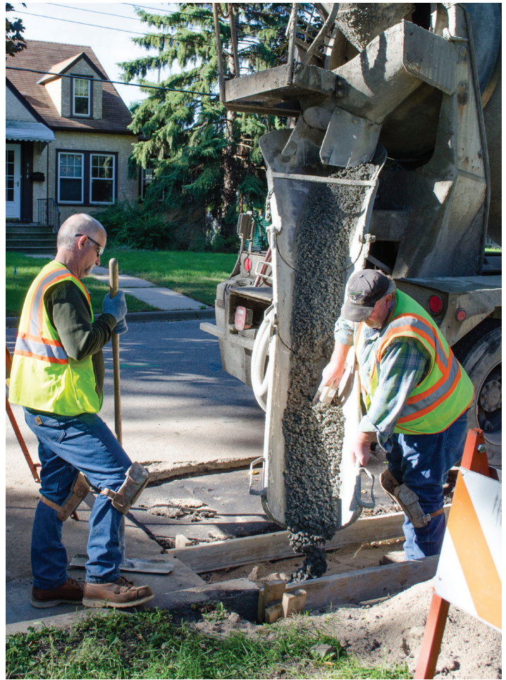
Curbs and gutters are replaced by restoration crews after work on an area is complete.
