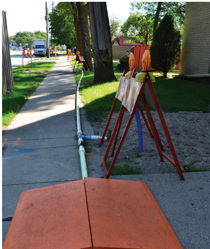
Temporary water mains line the sidewalk in areas of water main replacement.
