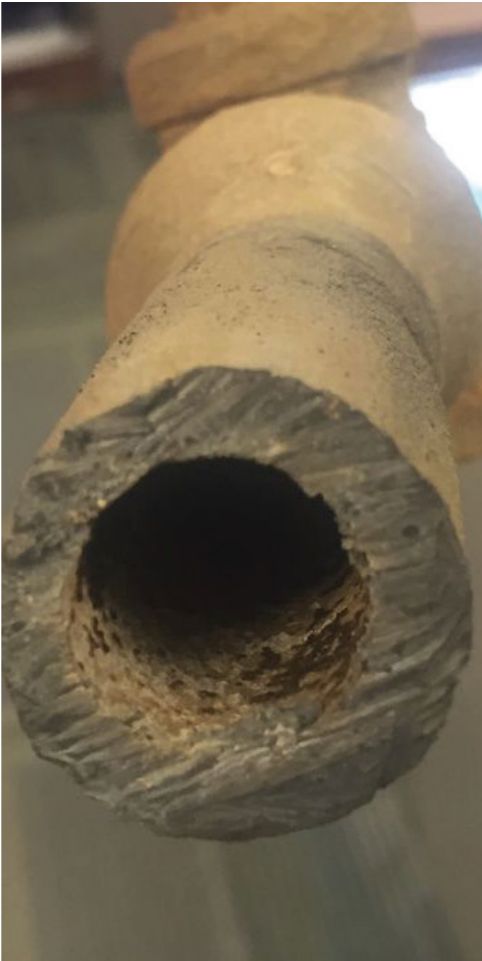
Lead pipes like this one throughout the SPRWS distribution system in service lines to older homes were the source of many communications efforts throughout the year.
