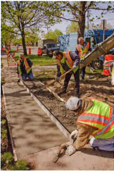
Above: Cement workers lay concrete to replace a sidewalk that was removed during water main replacement along Snelling Avenue in Saint Paul.
