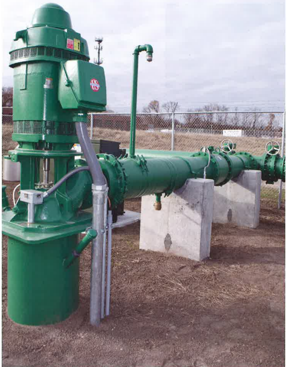
Above: Well I, one of 10 deep wells that act as additions to our main water supply from the Mississippi River. The 10 wells can supply the entire 45 million gallons a day used by the water utility on average should it be needed.
