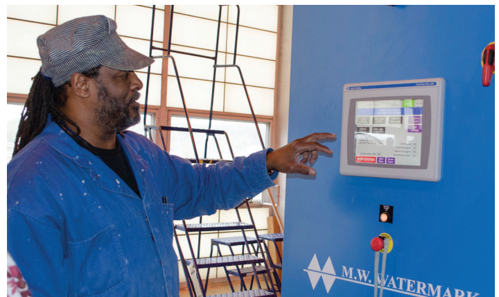
A worker uses a control panel on a dewatering press in the dewatering building.
