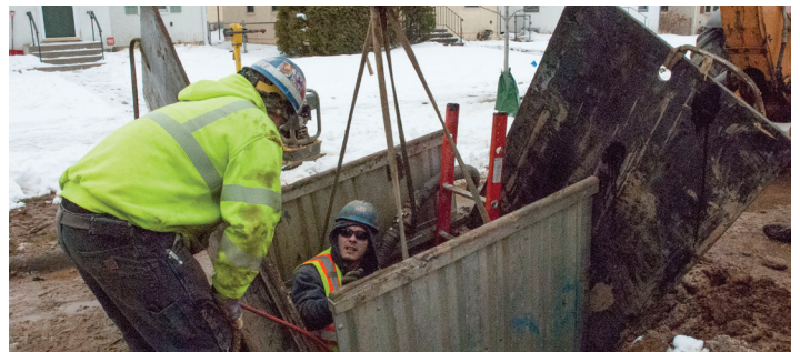
Workers fixing a small main break.
