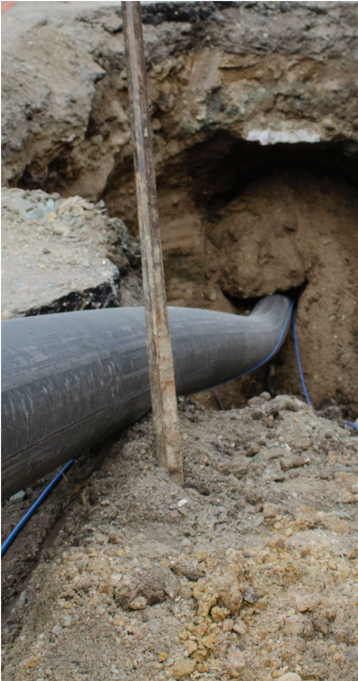
Pipebursting used to lay new main in residential areas.
