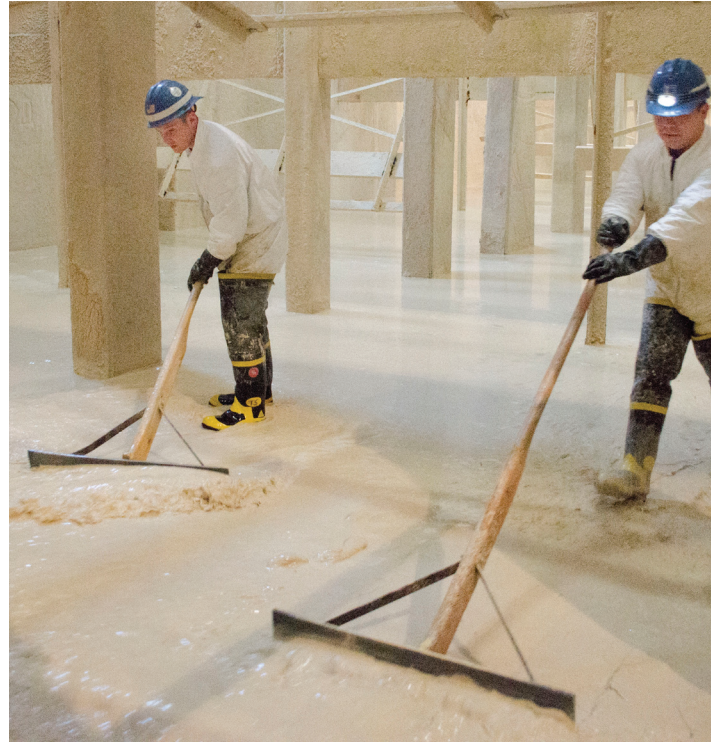
Workers clean out floc three in the plant.
