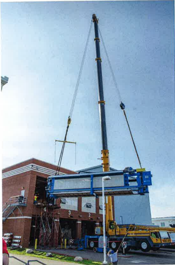
A new solids dewatering press (a filter press) was installed into the dewatering building to increase flexibility and redundancy to the waste removal process.
