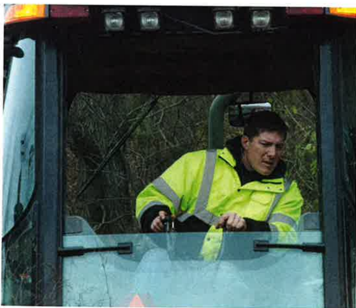
Distribution crews wrap up repairs on a leak (top), install new water main (center), and dig out a hole (bottom).
