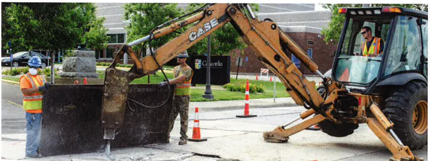
Opening the street to repair a main break.
