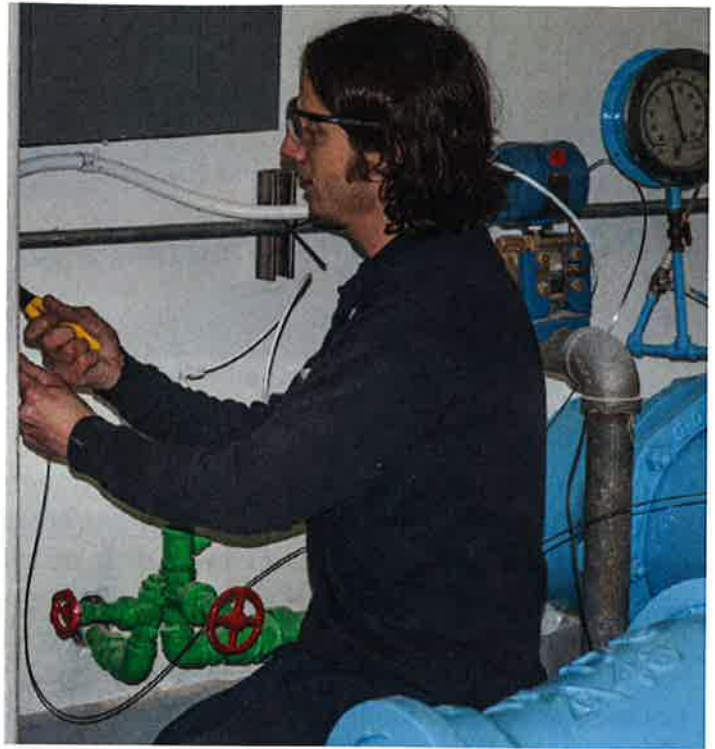
An electrician works onsite at a water tower.
