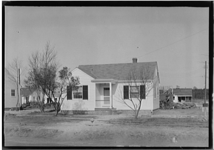
Figure 13 . Minimal Traditional FHA-Insured Home, 1941. Courtesy of the Library of Congress
