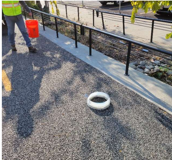
Photo 2-7: Permeable Pavement Infiltration Test
