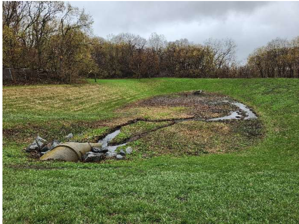
Photo 4-1: Bush Desoto in 2023 Before Reconstruction
