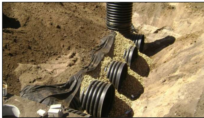
Photo 5-1: St. Albans 48” Perforated HDPE Installation
