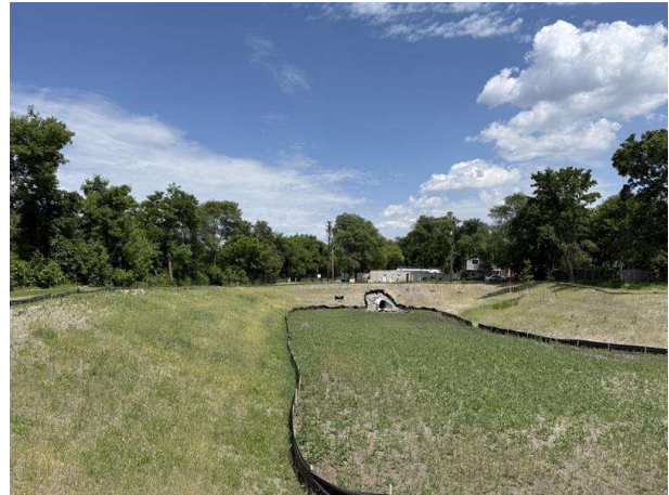
Photo 4-2: Bush Desoto in 2025 After Reconstruction
