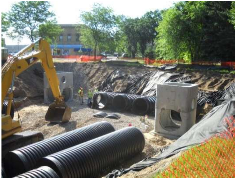
Photo 6-1: Hampden Park BMP Construction
