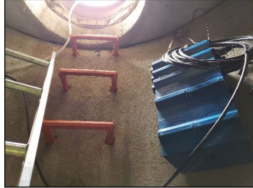
Photo 2-4: Flow Monitoring Equipment Install
