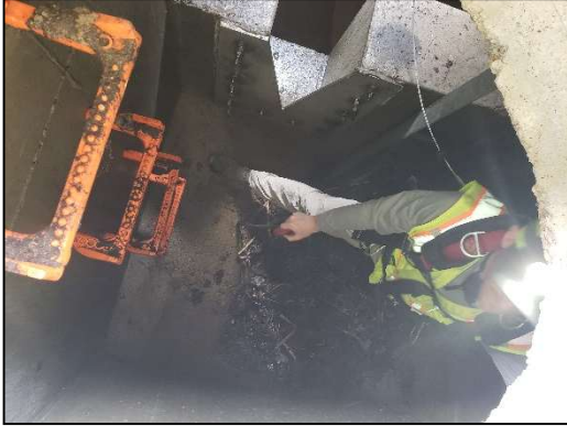
Photo 2-3: Flow Monitoring Module Install Process
