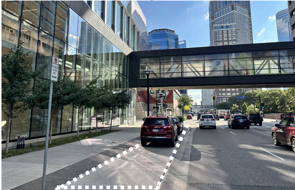
Figure 30 An example of a raised parking and loading area on 4th Ave S in Minneapolis
