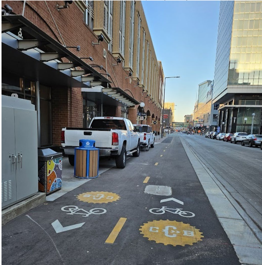
Figure 12 Trucks Parked Illegally Blocking Sidewalk and Capital City Bikeway
