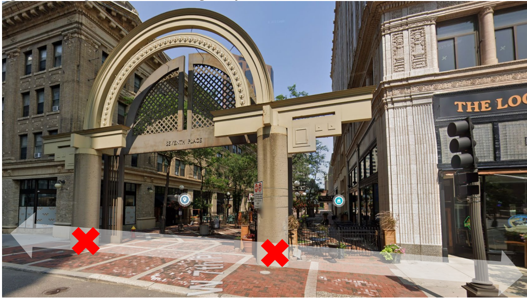
Figure 31 Existing view of the 7th Place gateway arch from St. Peter Street.
