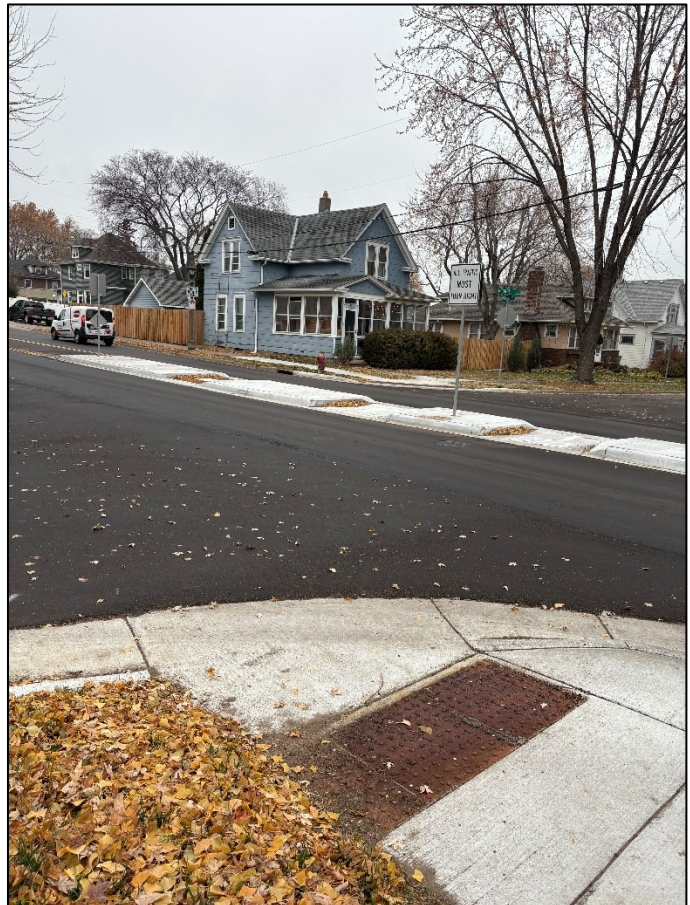
Example of Median Island
