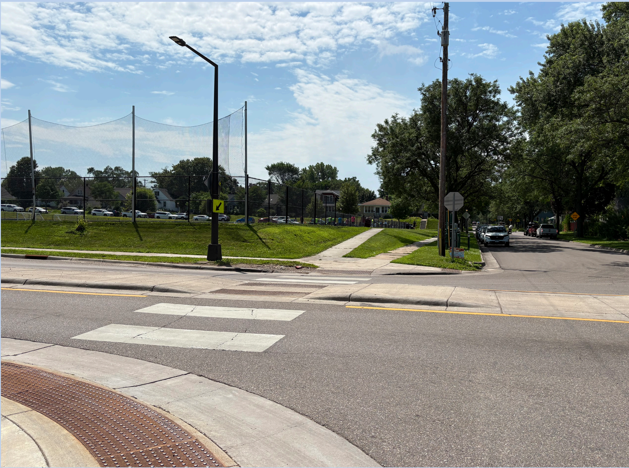
Maryland Avenue W and N Park Street in Saint Paul
