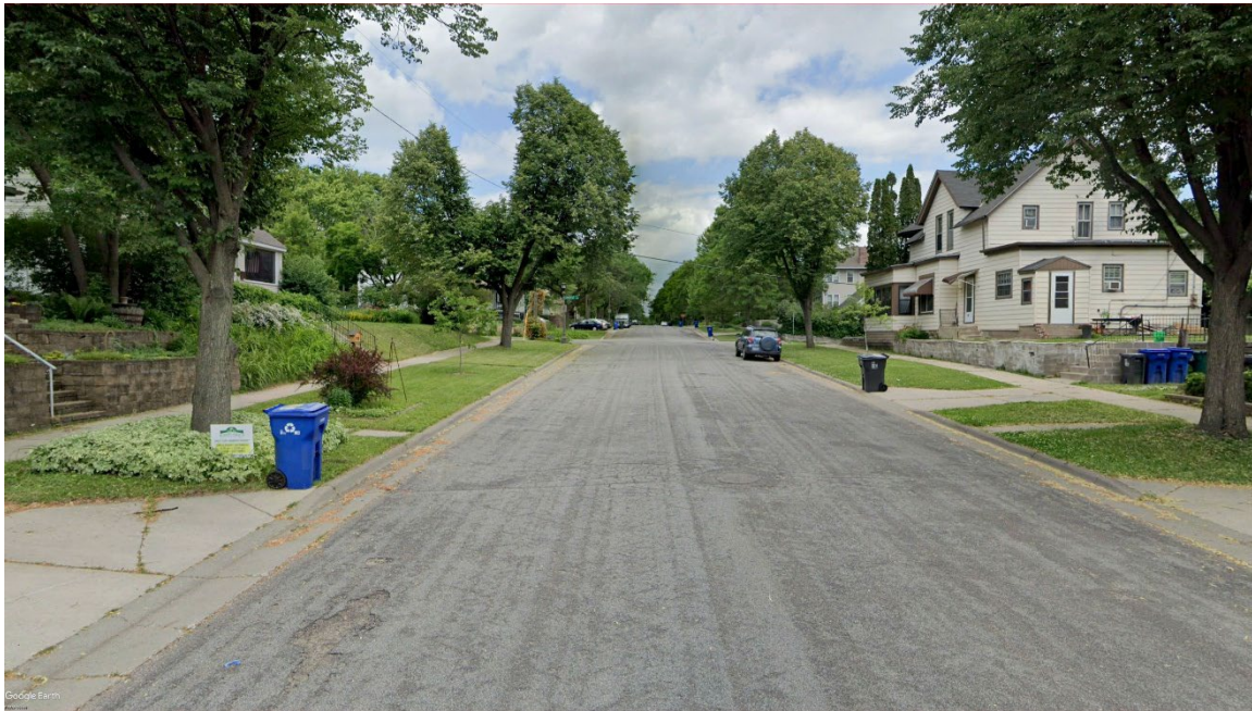
▲ Existing conditions on Hall Avenue between Winifred and Congress Streets.
