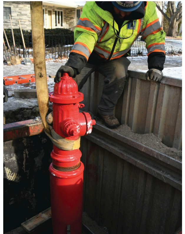
Installing a re-habbed original 1884 water hydrant.
